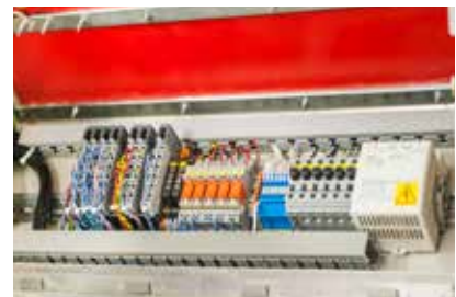
Advanced, PLC based control and DAQ electronics
